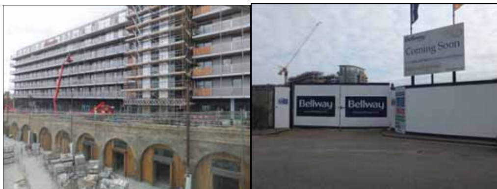
Photo 3.3: Kent Wharf construction site
